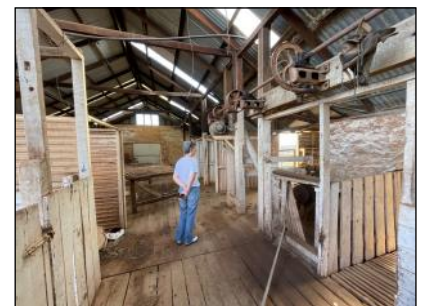
Derelict Bowes Estate shearing shed and homestead
