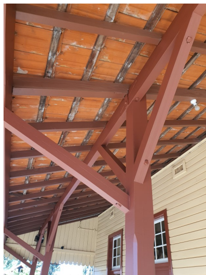
The finished beam structures of the station building
