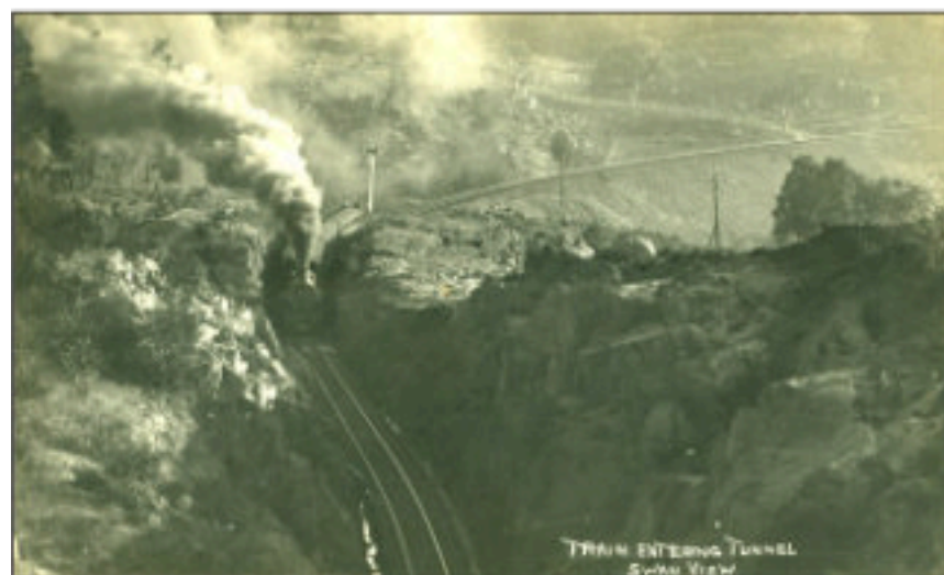
Swan View Railway Tunnel M1999.2381
